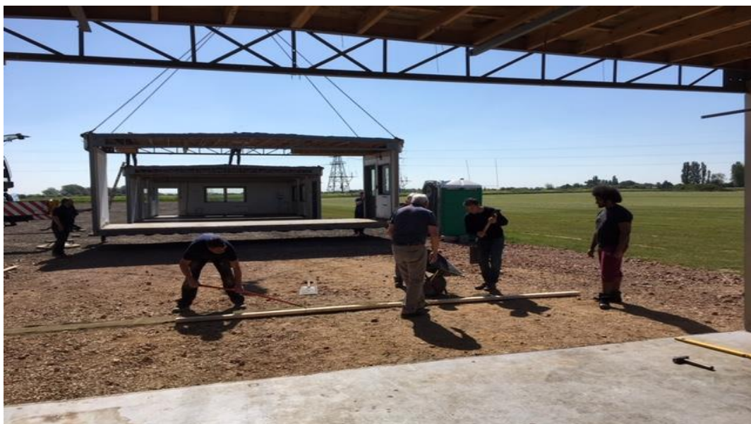
Crowland Cranes lifting the next Clubhouse bay into position with volunteers completing the foundations
